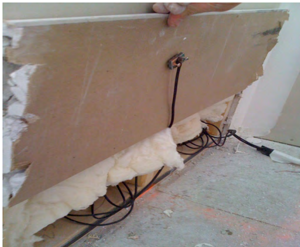
Figure 3. Installation of sensors on gypsum
